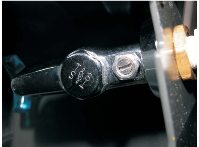
Water Flow Adjustment Screw
